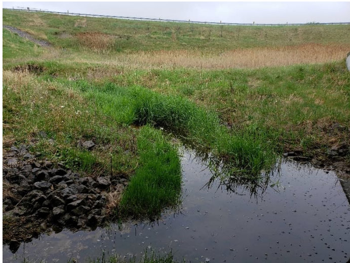
Photograph 183. ↑ C28-A-1, May 2022. Downstream reach facing downstream from culvert outlet.
