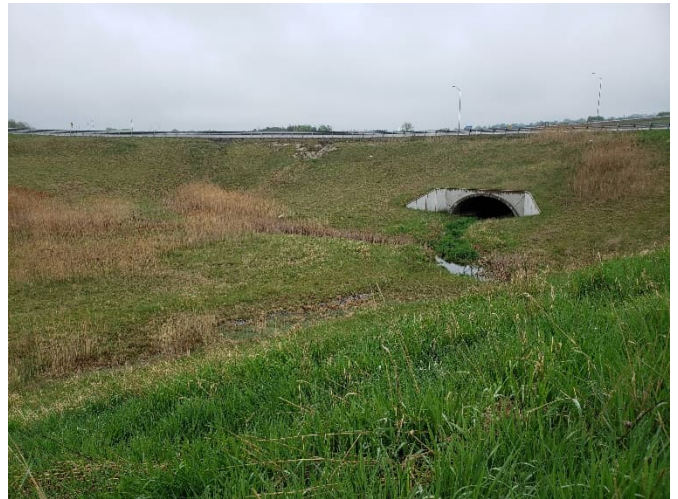
Photograph 180. ↑ C28-A-1, May 2022. Downstream reach facing upstream at culvert outlet.
