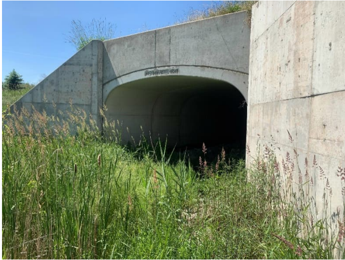
Photograph 173. ↑ C26-A-1, June 2021. Culvert outlet on east side of Highway 404.
