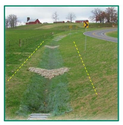
Figure 3A - Location of Permanent Flow Check Dams along a Flat Bottom Grassed Swale
