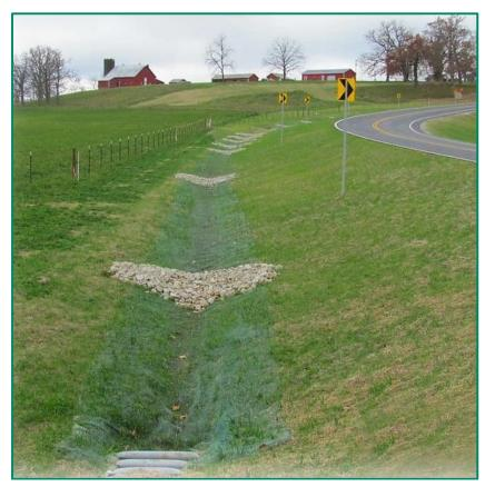
Figure 13: Location of the Flow Check Dams along a Flat Bottom Grassed Swale
