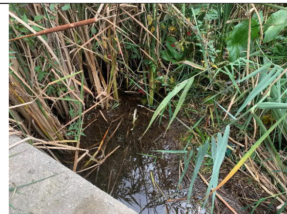
Photograph 11: County Road 4 culvert outlet looking west. Dense phragmites immediately downstream.
