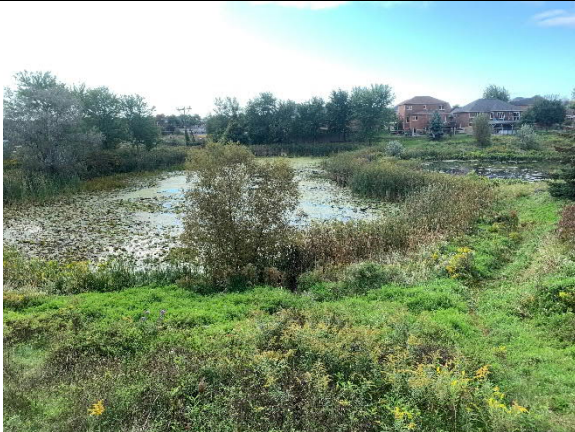
Photograph 3: SWMP forebay and detention pond, looking south from earth berm.
