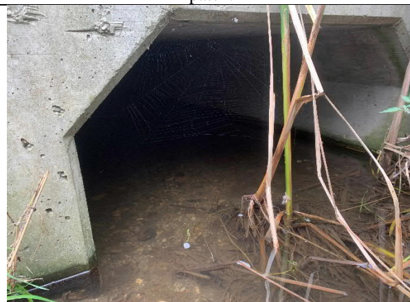
Photograph 12: County Road 4 culvert outlet.
