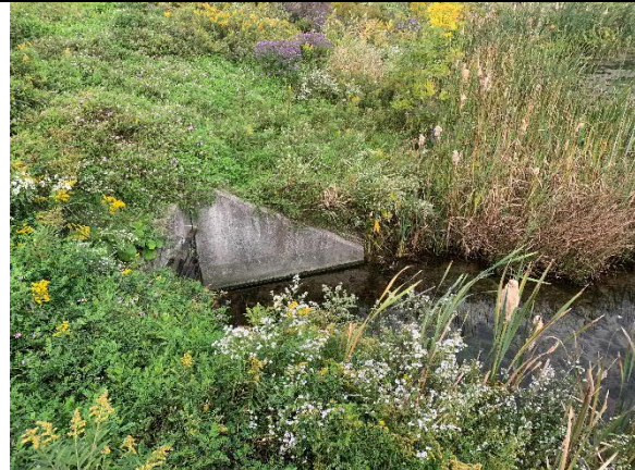
Photograph 2: SWMP inlet at southwest corner of pond forebay.
