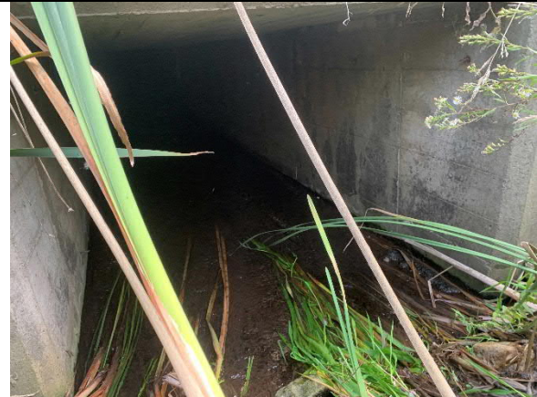
Photograph 8: County Road 4 culvert inlet, laminar flow across concrete bottom.
