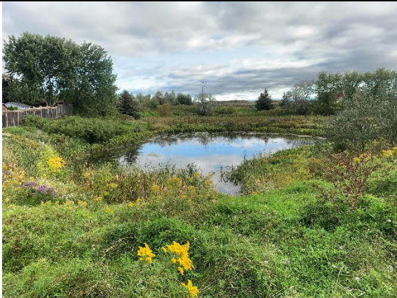
Photograph 1: SWMP forebay, looking north.
