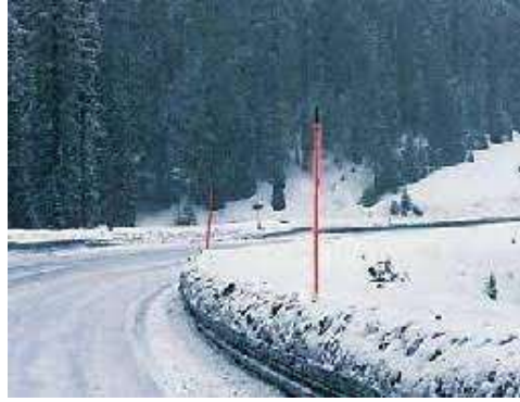
Figure 33 Pavement edge marker with reflector
